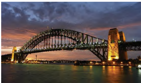
(ก) Sydney Harbour Bridge, Australia [1]
